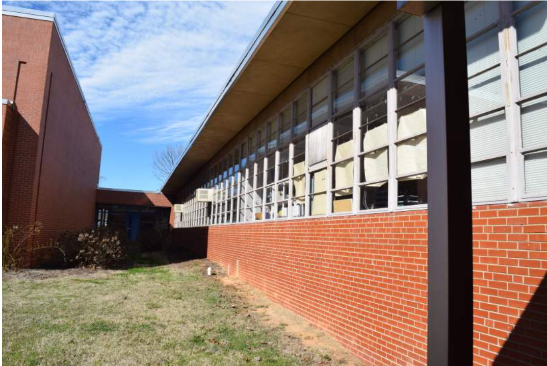
Figure 25: Rear of 1965 building, view to the northwest
