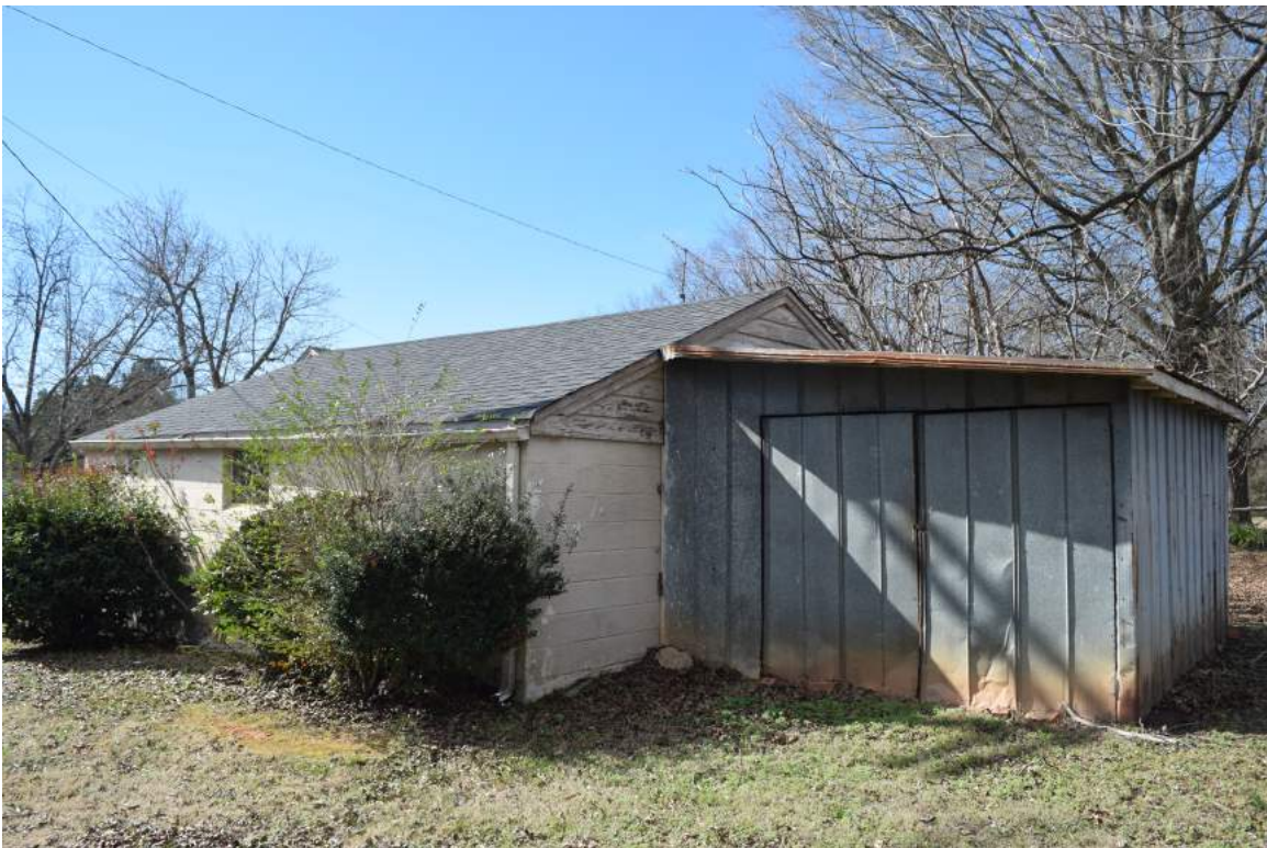
Figure 11: Concrete block garage and attached metal shed, view to the west-southwest
