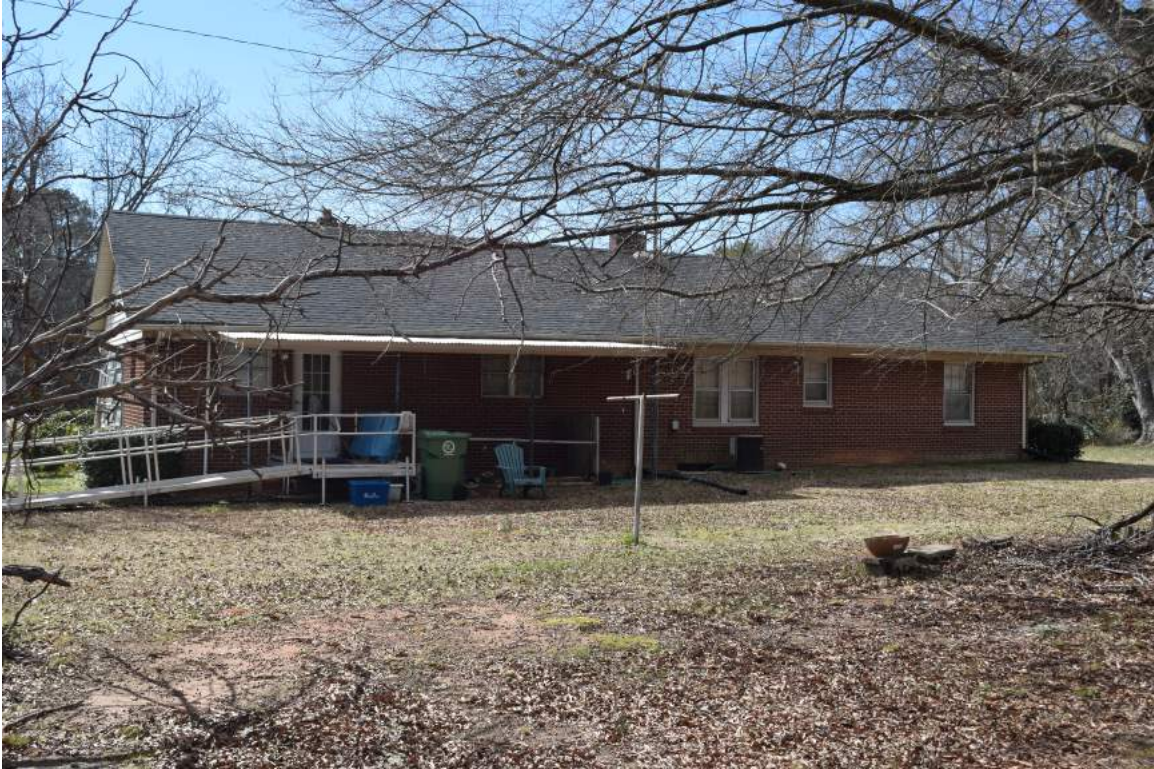
Figure 10: North (rear) elevation, view to the south
