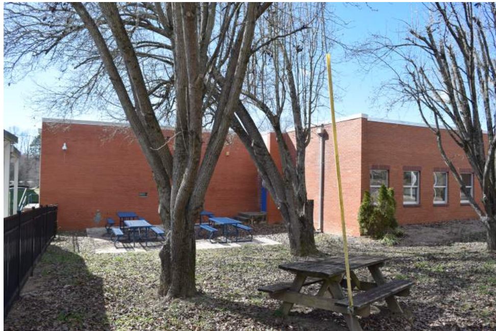
Figure 28: ca. 1980 addition on south end of building, view to the southwest
