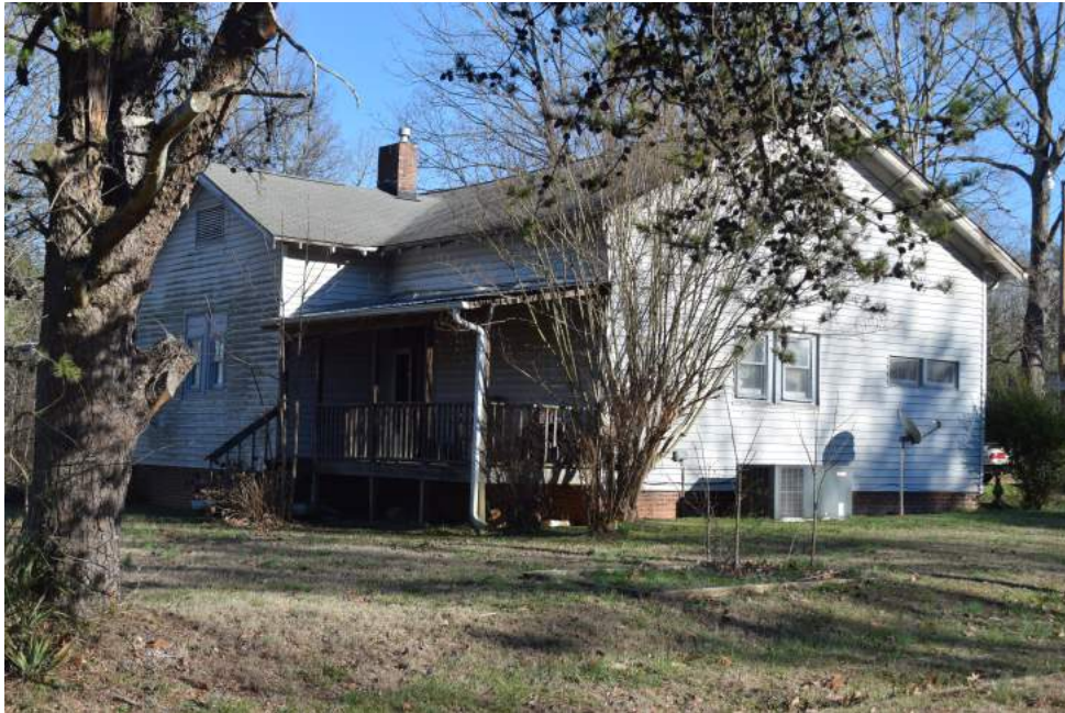
Figure 81: Northwest corner of Beaver Dam School, view to the southeast
