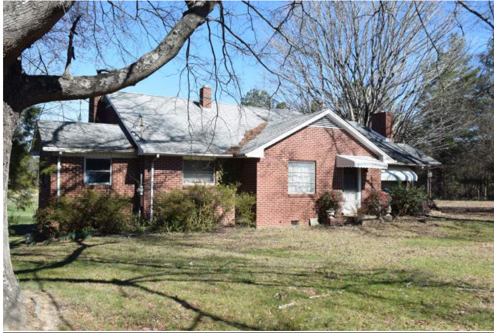
Figure 50: Mauney House facade, view to the northeast
