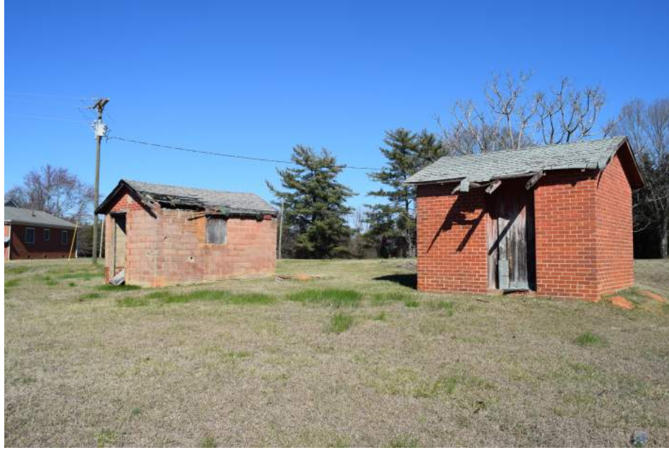
Figure 31: Outbuildings north of Southern Machine Company building, view to the north
