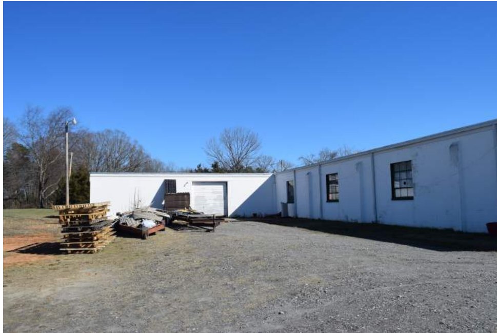
Figure 33: 1960s addition on the north side, view to the east
