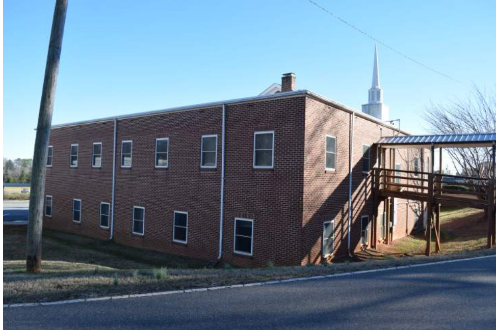
Figure 72: Rear of education building addition, view to the southeast
