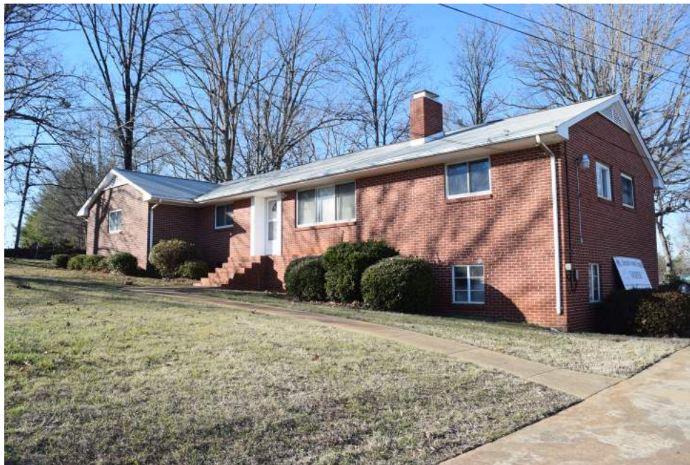
Figure 75: Parsonage, view to the northwest
