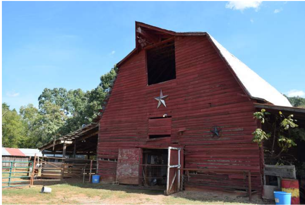
Figure 58: Cattle barn built in 1911, view to the northeast
