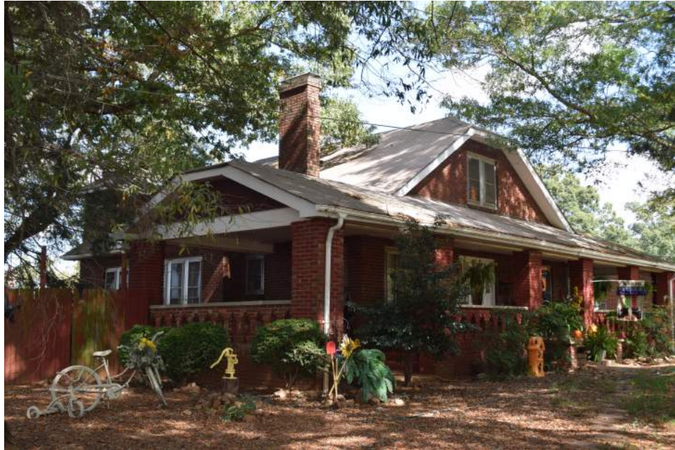
Figure 55: Forrest Allen House, southwest corner, view to the northeast
