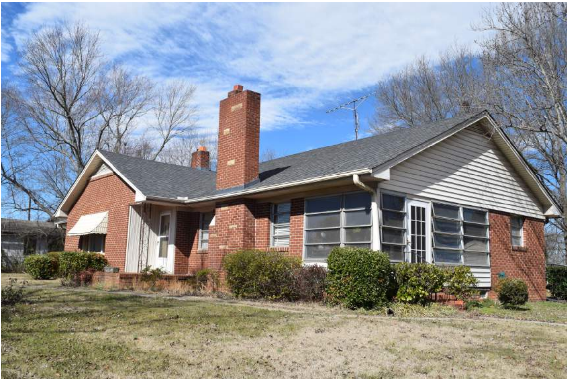
Figure 9: southwest (front) corner, view to the northwest
