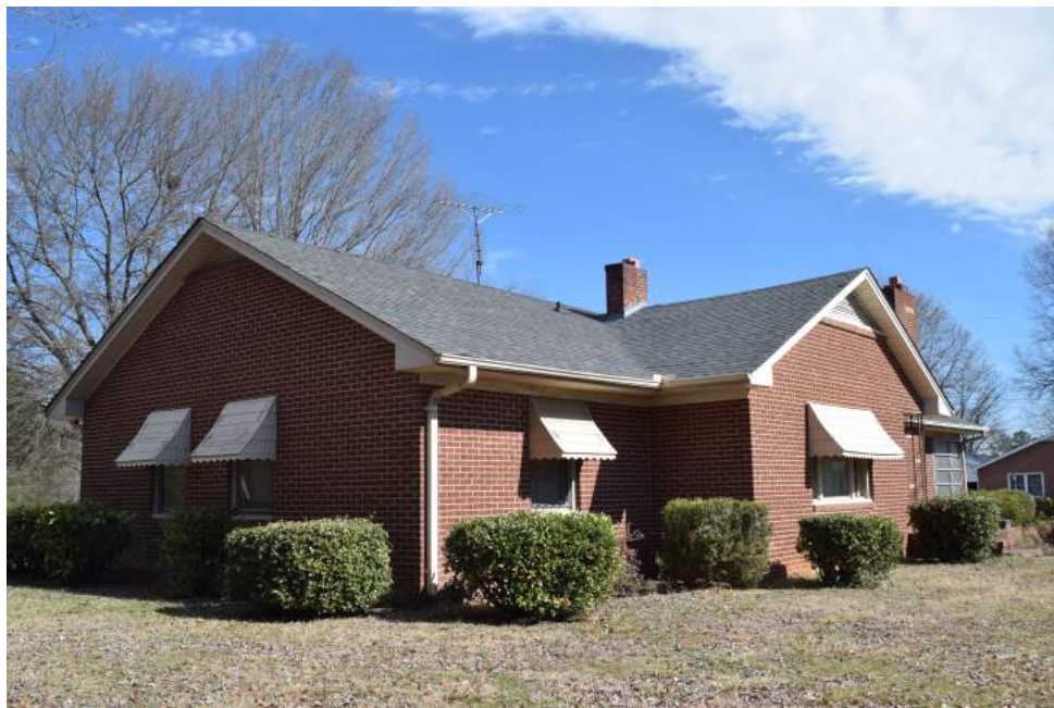
Figure 13: Best House southwest corner, view to the northeast
