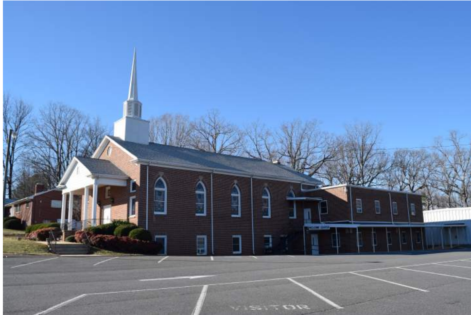
Figure 71: Mount Beulah Baptist Church, original church, education building, addition, and modern metal building (left to right), view to the northwest (parsonage partially visible to the left)
