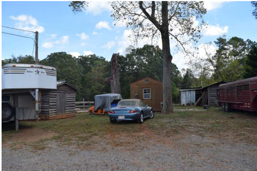
Figure 61: Well house, modern storage building, and smokehouse (left to right), view to the east
