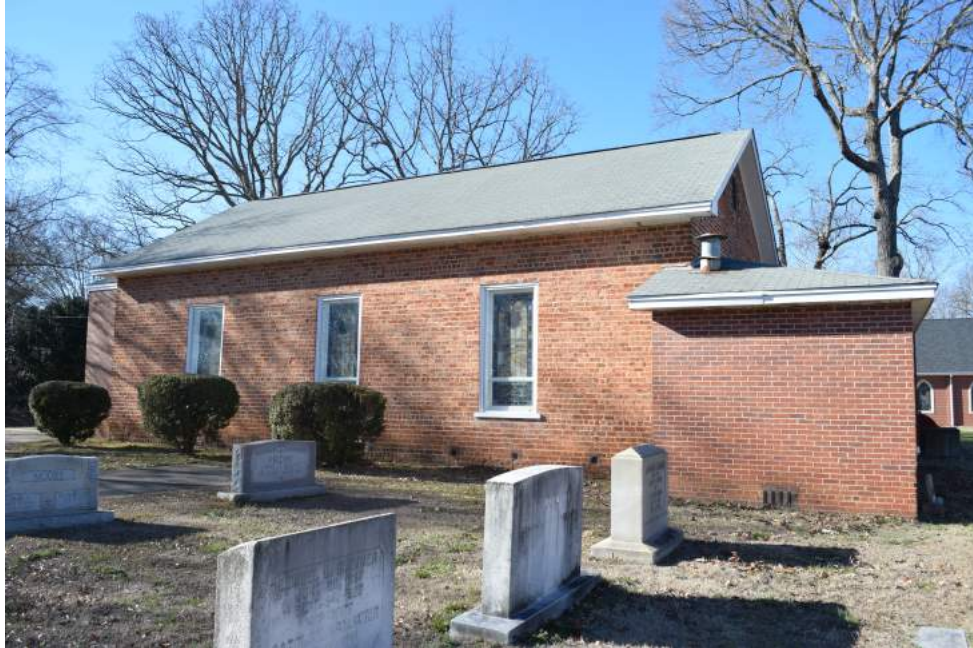
Figure 15: 1883 church with 1939 rear addition, view to the northwest
