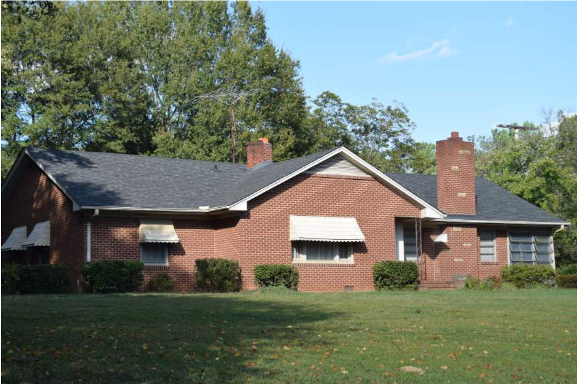
Figure 7: Facade (south elevation) of house, view to the north
