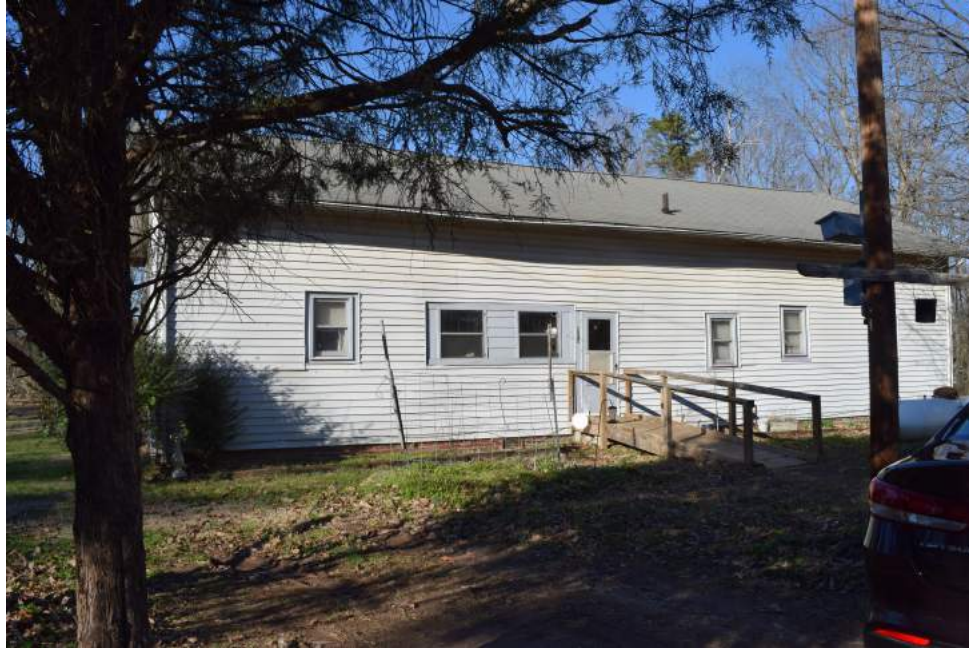
Figure 79: Beaver Dam School, rear elevation, view to the northeast
