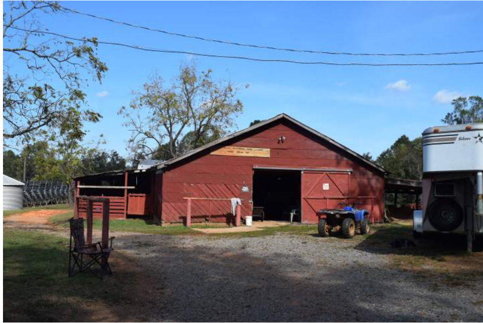
Figure 60: Barn built in 1936, view to the north
